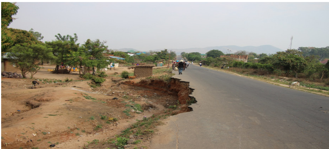
Photo 3. National road N°5 in SANGE in a state of disrepair due to erosion
