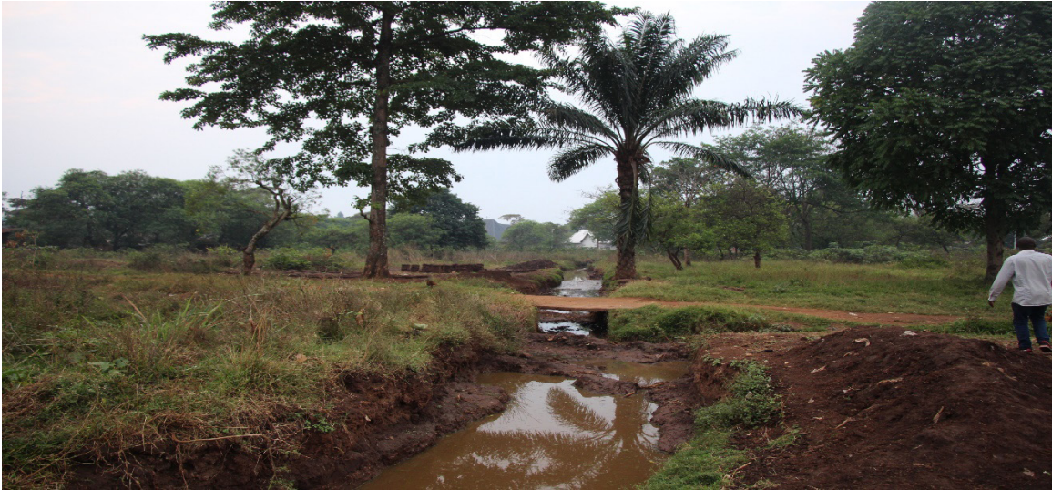
Photo 1: Emergency canal built by the population in LUVUNGI to evacuate the water that causes flooding in the neighbourhoods
